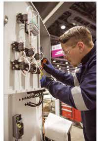
Tyrone Bunce wiring the panel.
