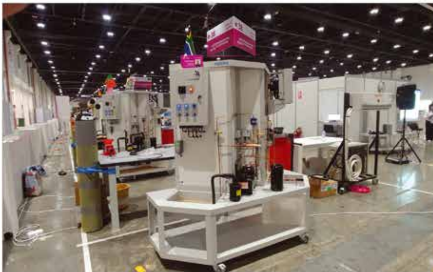
Tyrone Bunce "2017 Worldskills Project Plant" completed in given time and working according to given specification.
